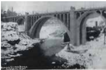
January 1912 — Completed structure representing the largest single masonry arch in the United States.
