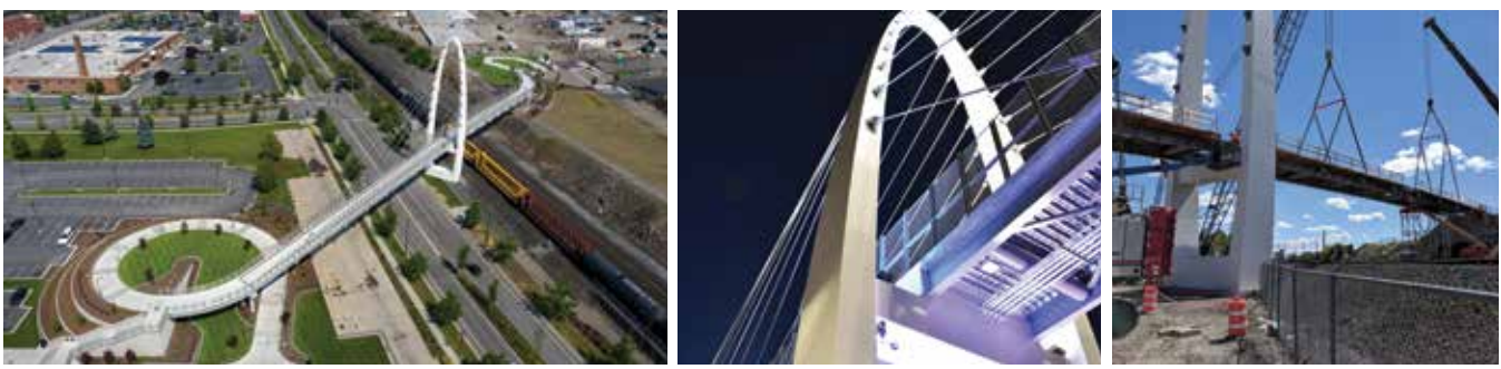
Photos by Garco Construction and KPFF Consulting Engineers.
