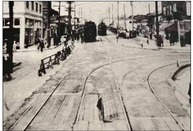
Warren Wing The Junction, looking north on California Avenue, March 18, 1926. Paving of the intersection with brick had just been completed when this photograph was taken.
