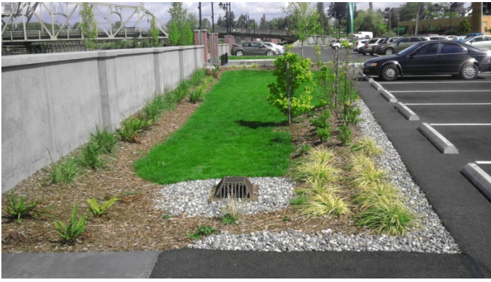
Left: Bioretention LID cells improve water quality running off of the parking lot.
