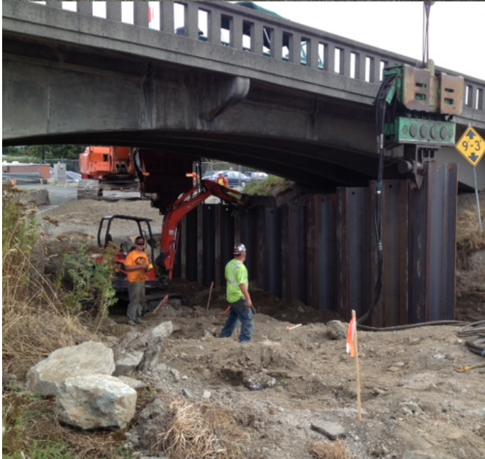
Top: Sheet piling installation near Commercial Cold Storage (CCS). Middle: Complete and exposed sheet piling by CCS. Bottom: Workers install sheet piling underneath the Division St Bridge (SR536).
