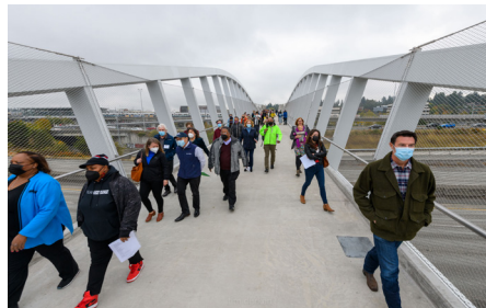
Crossing I-5 on the Vierendeel truss span
