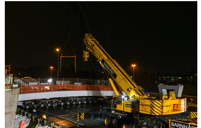
Thru-girder installation using SPMT transporter during I-5 closure
