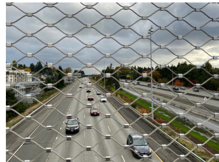
Transparent cable netting functions as a safety barrier and provides an unobstructed view
