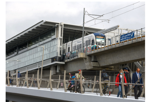
Ramps with 8 percent slopes have landings for all types of non-motorized travelers
