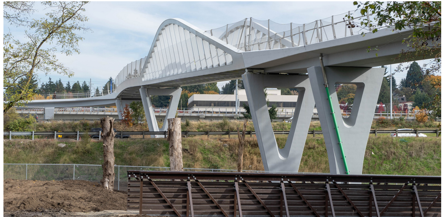
The bridge's Vierendeel truss, thru-girder, and pre-cast girders span I-5 and adjacent wetlands
