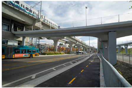
Multimodal transportation connections at terminus of bridge
