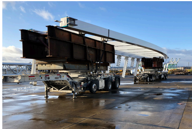
Transporting sections of the Vierendeel truss
