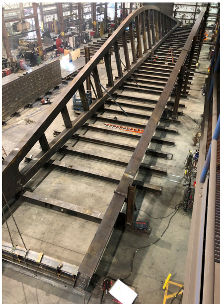
The Vierendeel Truss during fabrication
