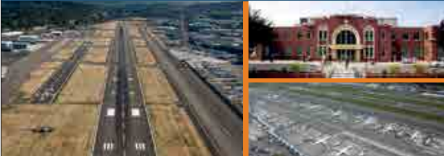
Boeing Field, King County International Airport (Seattle, WA)
