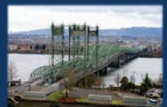
Columbia River Interstate Bridge Portland to Vancouver (1917)
