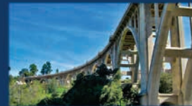
Arroyo Seco Bridge in Pasadena, California (1913)
