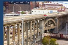
Twelfth Street Bridge in Kansas City, Missouri (1915)
