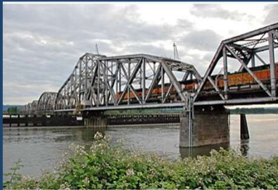
A train crossing the bridge's 467-foot (142 m) swing-span section
