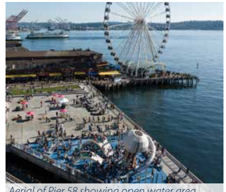
Aerial of Pier 58 showing open water area adjacent to seawall looking south.
