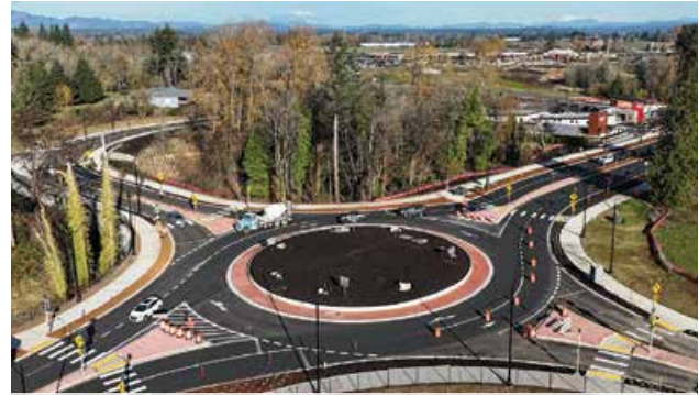
Completed 50th Avenue roundabout with final pavement and striping.
