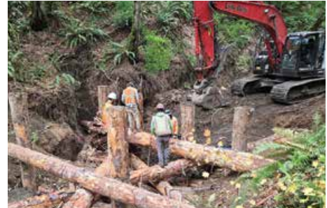
Log jam construction.
