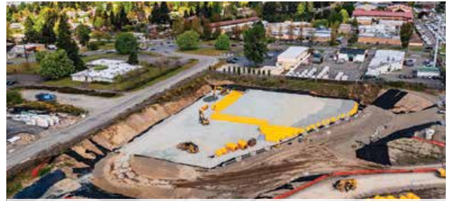
Aerial view of project site during installation of infiltration chambers, May 2024.
