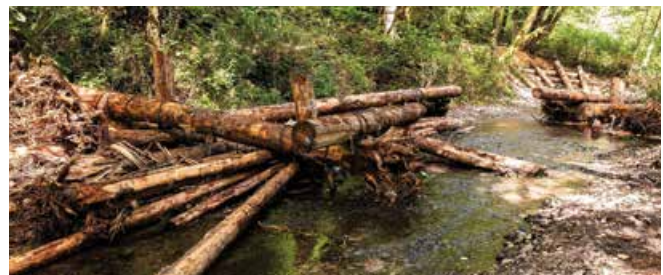
Engineered logjams - Site 1 downstream reach.
