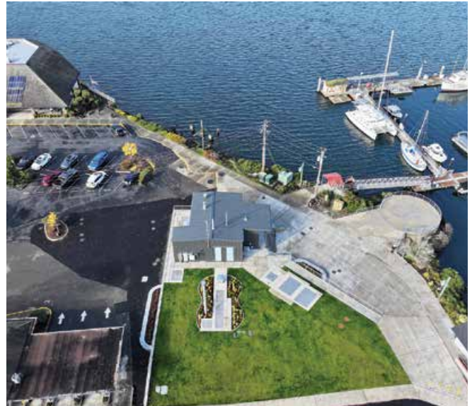
The fully completed pump station showcases its elevated superstructure designed for climate resilience.
