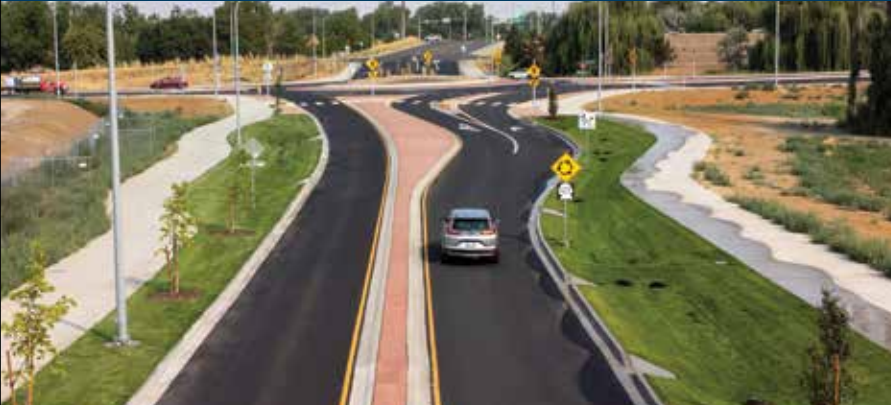
Myra Road South Extension Project Photo Courtesy of the City of Walla Walla
